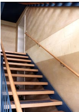
Staircase walls made of unfired earth bricks. The reverse side of the earth brick walls help regulate the moisture content of the air in the bathrooms.
