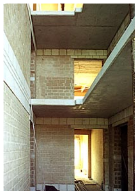
Staircase walls made of unfired earth bricks. The reverse side of the earth brick walls help regulate the moisture content of the air in the bathrooms.
