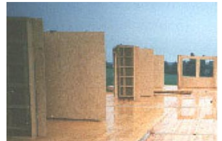
Solid wood strip ceiling elements
