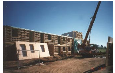
Erection of prefabricated panels
