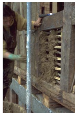
Repairing earthen infill panels Haus Schneiker
