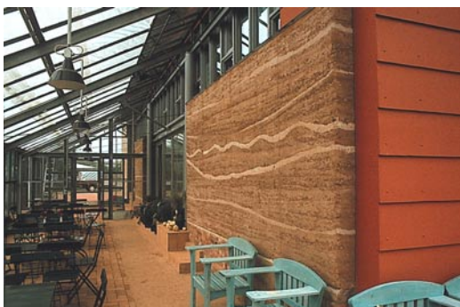
Coloured striations in the rammed earth
