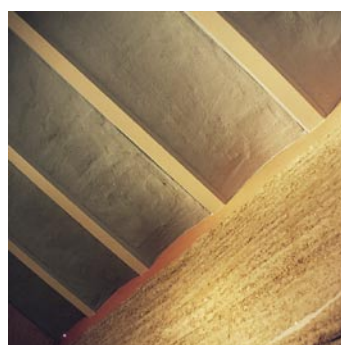
Junction between earth wall and ceiling
