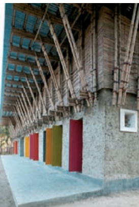
Corner detail showing earthen and bamboo construction
