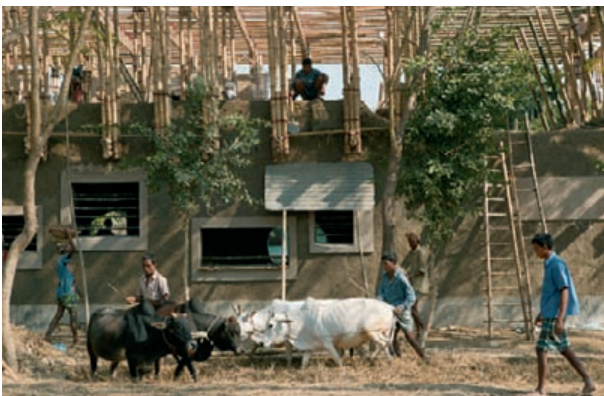
Cows help mix the earth, water and rice-straw mixture
